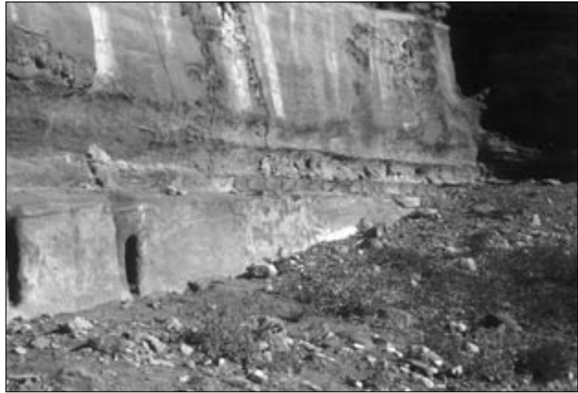
Figure 6. Dual pipelines continuing past the theatre to supply tanks (T) above the Cardo .
