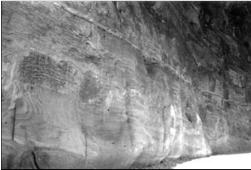
Figure 3. Elevated water channel/piping system on west face of El Khubtha Mountain.
